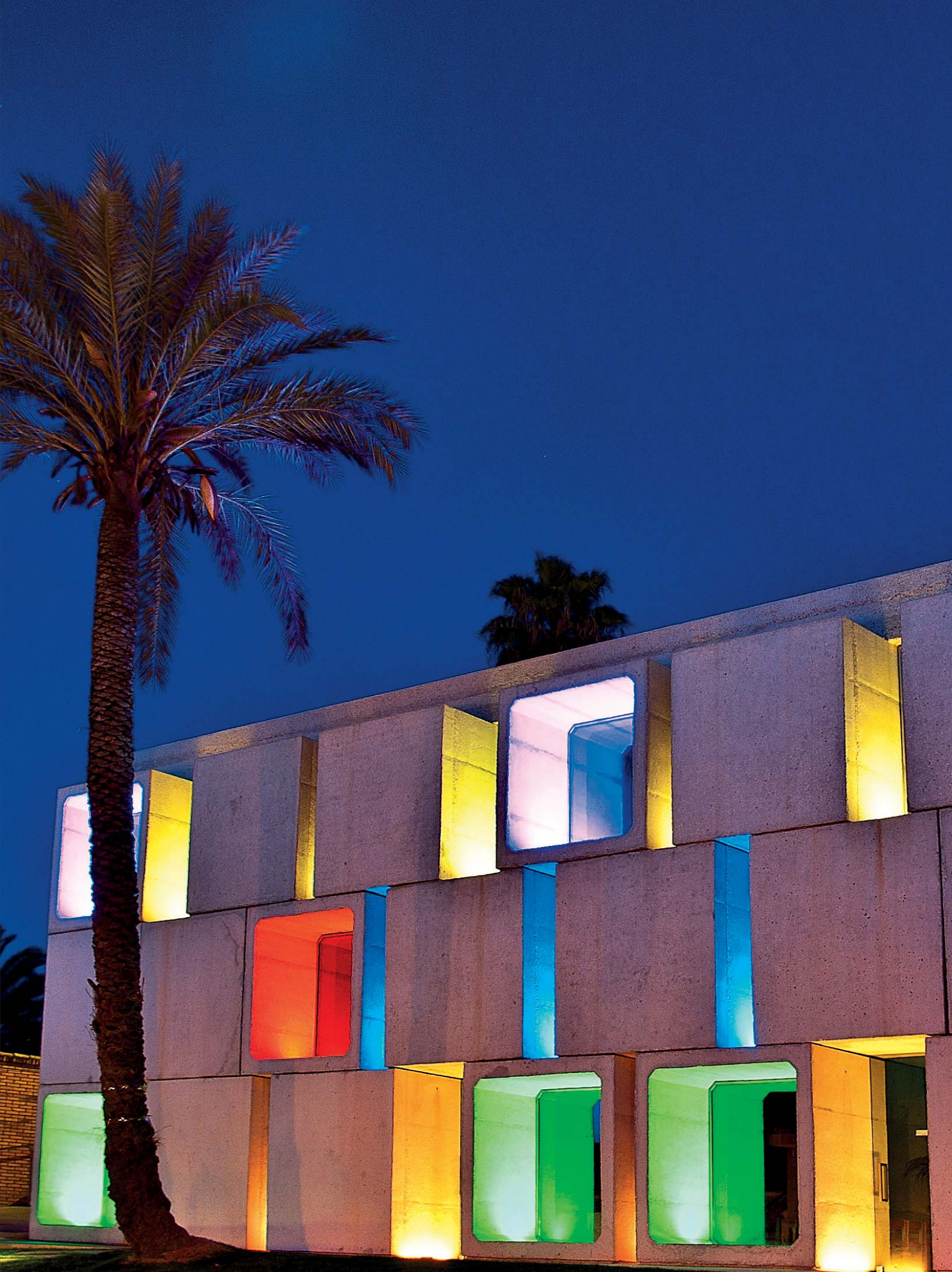
Biblioteca Antonio Gala - Guadalcazar, Spagna - Tekno RGB - Arch. Francisco Lopez Redondo - Lighting Designer Jose Benitez - Foto Salamanca Antonio Gala Library - Guadalcazar, Spain - Tekno RGB - Arch. Francisco Lopez Redondo - Lighting Designer Jose Benitez - Photo Salamanca
