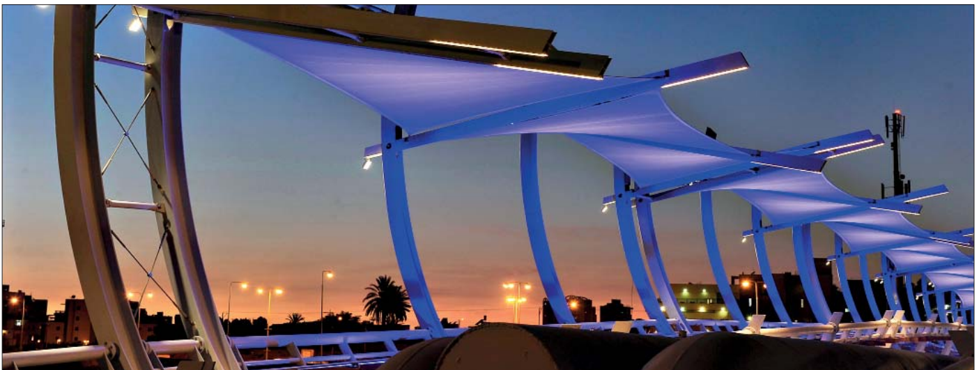
Pipe Bridge - Be'er Sheva, Israele - Tekno 3W 3000K - Arch. Rami Marash - Lighting Designer Amir Brener Pipe Bridge - Be'er Sheva, Israel - Tekno 3W 3000K - Arch. Rami Marash - Lighting Designer Amir Brener
